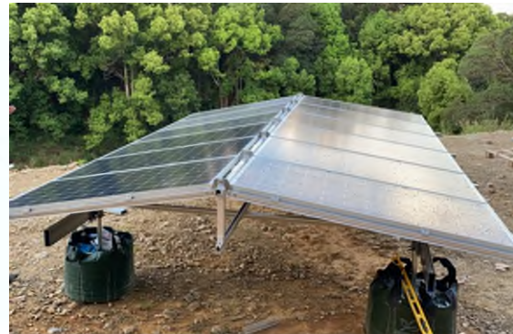
Figure 65 - Solpod Ground ballasted steel frame pod
