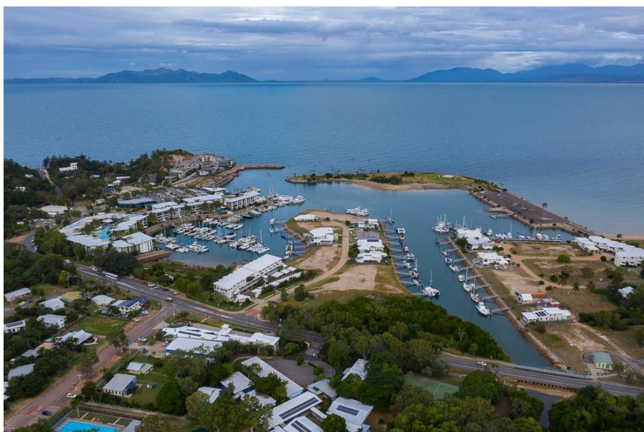
Figure 1. The completed Nelly Bay marina on Magnetic Island.
